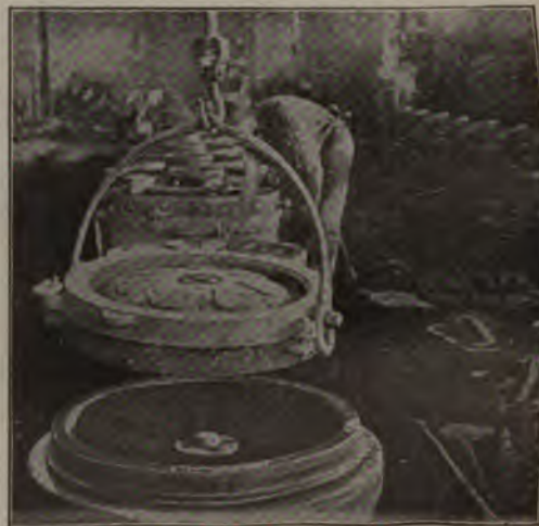
OPENING THE MOLDS.
